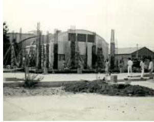
Pakistan Cables Factory SITE, Karachi
