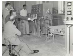
Aluminium Rod Extrusion Plant installed
