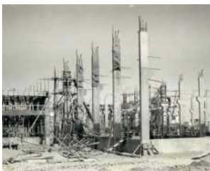
Expansion of Factory took place for manufacturing of power cables
