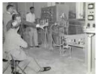
Aluminium Rod Extrusion Plant installed
