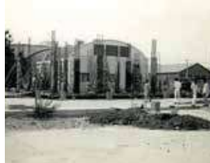
Pakistan Cables Factory SITE, Karachi
