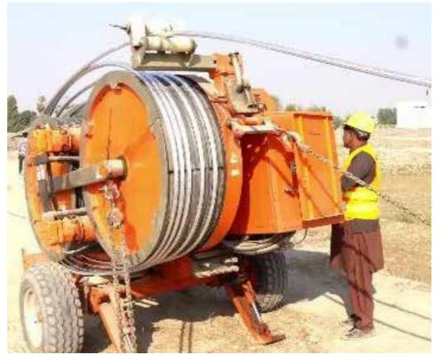
With the re-conductoring of the existing AAAC Greely Conductor to the Pakistan Cables ACCC® Drake Conductor the capacity of transmission line increased from 1800 Amps to 3200 Amps. In addition, the Sag Profile of transmission has been improved, which is a major relief for the residents residing in the buildings under the transmission line. The clearance of line from residential buildings has improved significantly and without any modification in the existing structures and right of way problem.
